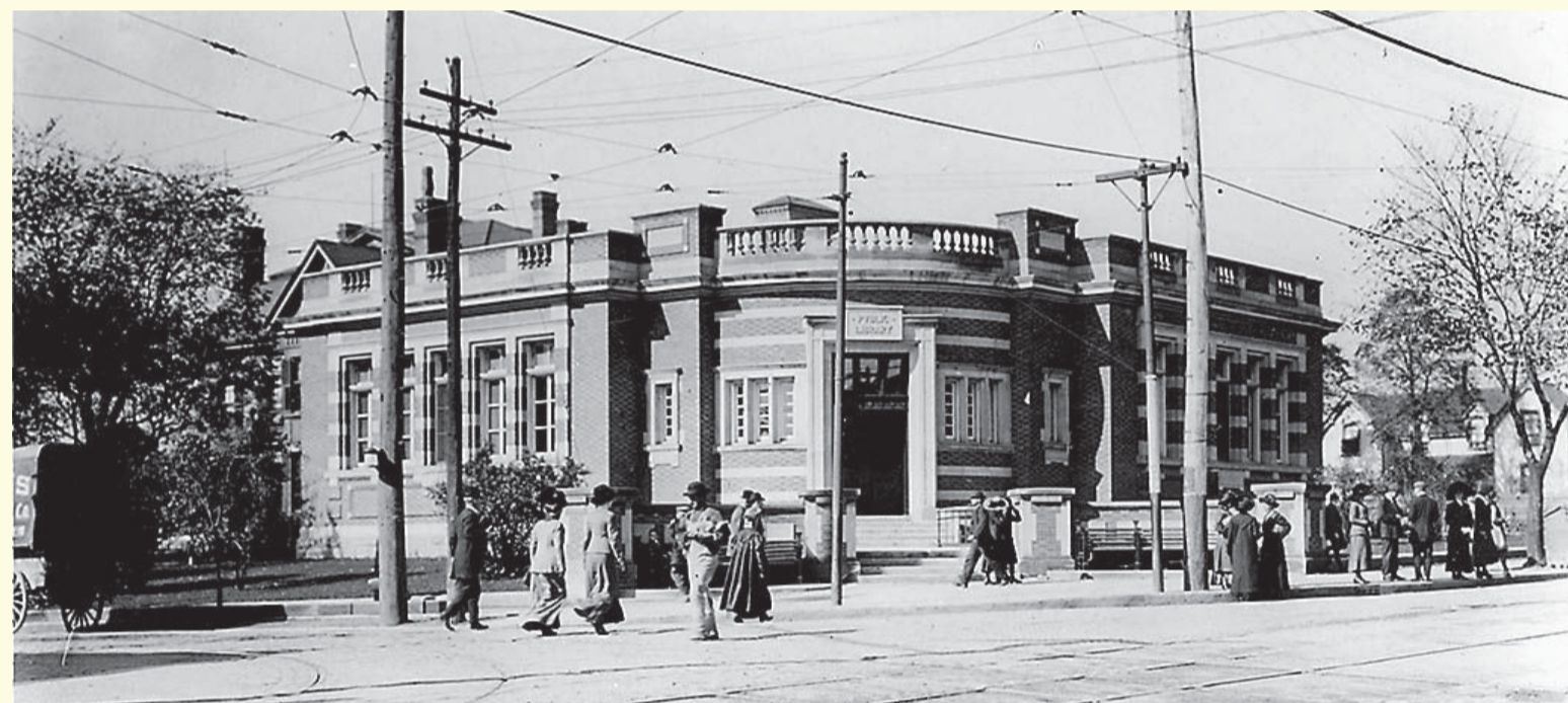
Riverdale Branch, about 1911 Designed in a Georgian Revival style by city architect Robert McCallum, the branch was constructed of red brick with white Ohio sandstone trim at a cost of $24,174. It featured a distinctive upper balustrade, a retaining wall in matching materials, and, rare for a Carnegie library, a corner entrance. Note the benches in front of the wall installed in 1911 with funds provided by the Riverdale Business Men's Association.
