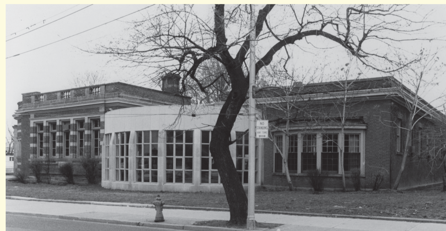
East facade showing the 1910 building (on the left) and additions from 1927-8 (right) and 1979-80 (middle), 1980
